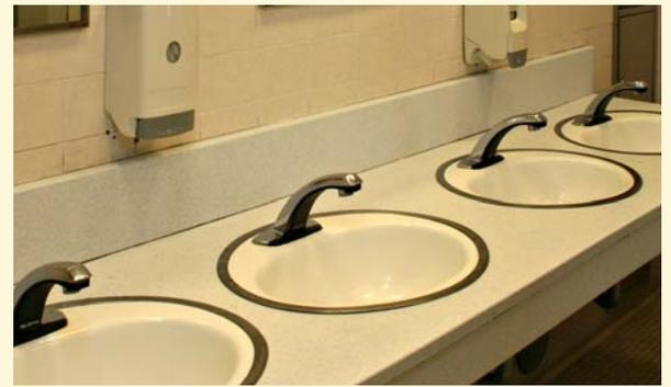
*New low-flow, infrared sensor-type lavatory faucets were installed in Murchison Gym. New ultra-low-flow urinals were also installed.*
