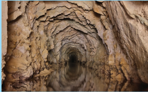
Doulton Tunnel, a horizontal well, source of groundwater and conveyance from Jameson Lake.
