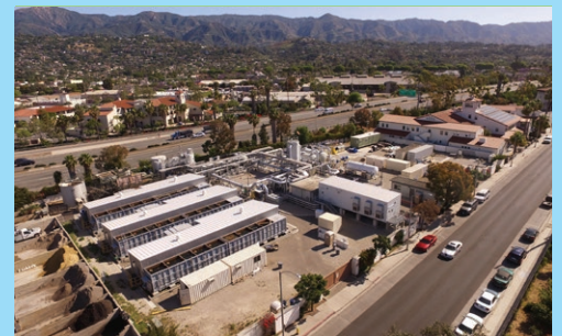
Water Supplied by the City of Santa Barbara, secured by Charles E. Meyer Desalination facility.
