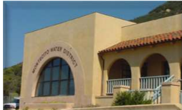
Bella Vista Treatment Plant
