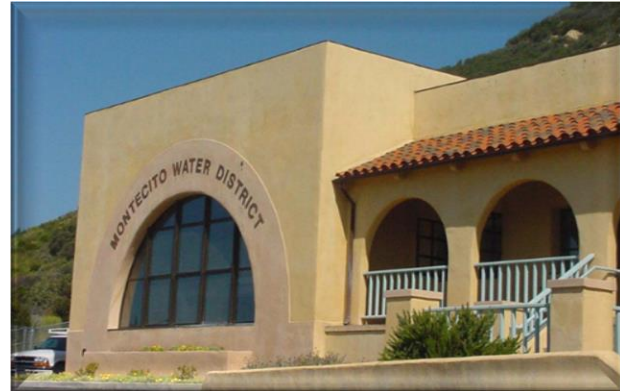
Bella Vista Treatment Plant
