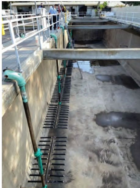
Photo 3.26 Air Diffuser System
