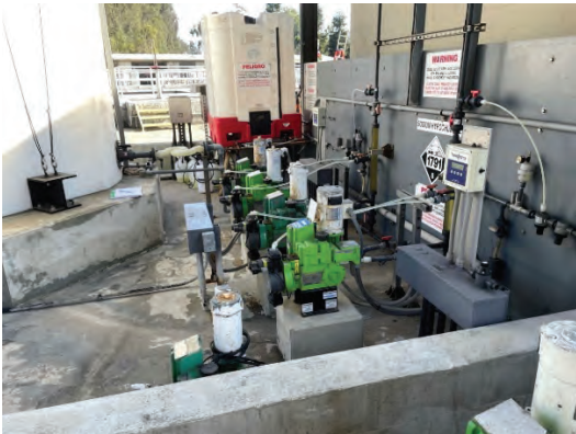
Photo 3.35 Sodium Hypochlorite Storage Facility
