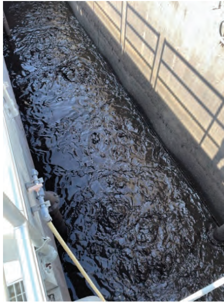
Photo 3.42 Aerobic Digester
