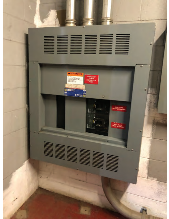
Photo 3.14 Emergency Distribution Panel
