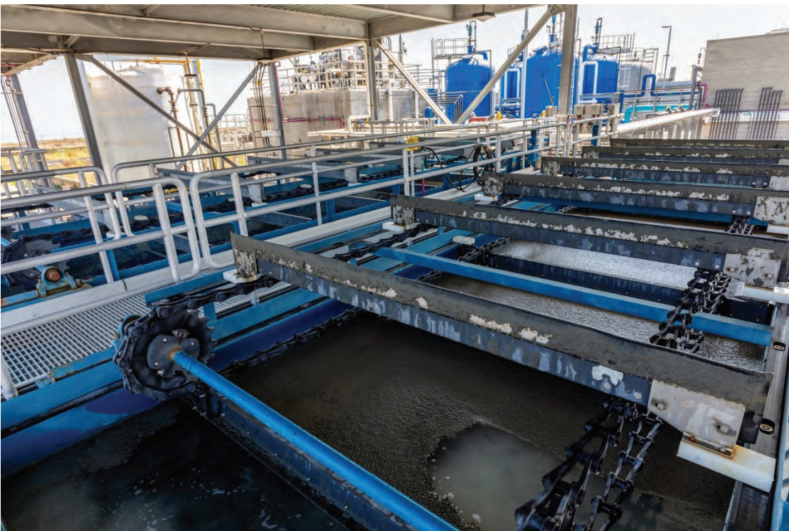
Figure 7.7 DAF Unit in Service
