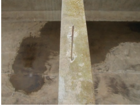
Photo 3.21 Aeration Basin 2 Exposed Rebar
