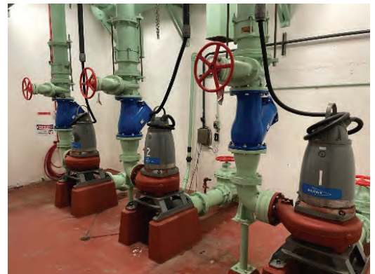
Photo 3.8 Influent Pumps/IPS Pump Room (Basement Level)
