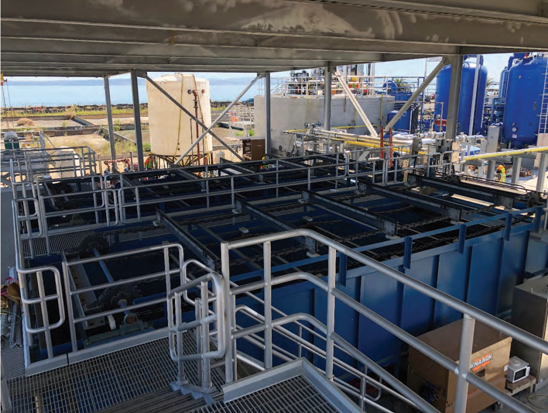
Figure 7.6 DAF Unit Sludge Scraper System
