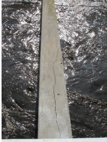
Photo 3.17 Aeration Basin 1 Strut Cracking
