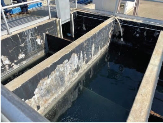
Photo 3.33 Chlorine Contact Basins
