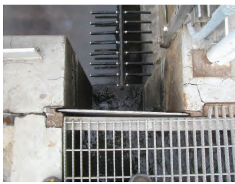
Photo 3.24 Aeration Basin 2 Channel Gate
