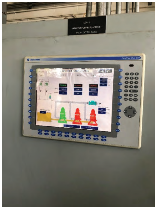
Photo 3.11 IPS Control Panel
