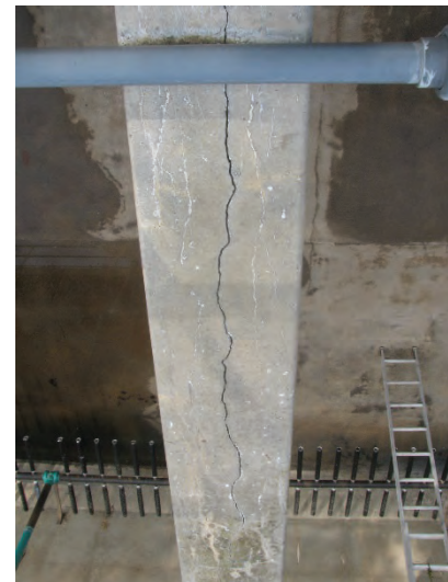
Photo 3.20 Aeration Basin 2 Cross Beam Longitudinal Cracking
