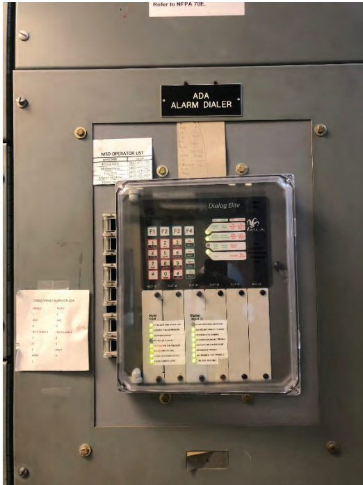
Photo 3.49 Old Control and ADA Alarm Panel
