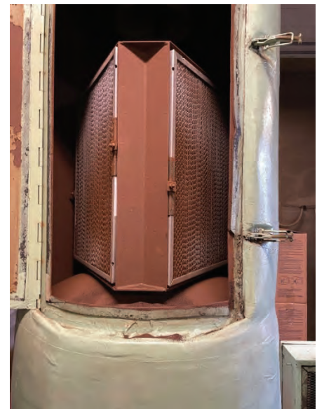
Photo 3.32 Aeration Basin Filter Silencer
