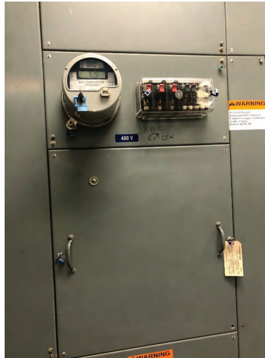
Photo 3.50 Service and Metering Cabinet
