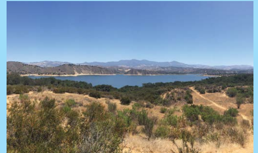
Cachuma Project (Lake Cachuma), a federally owned surface water facility.
