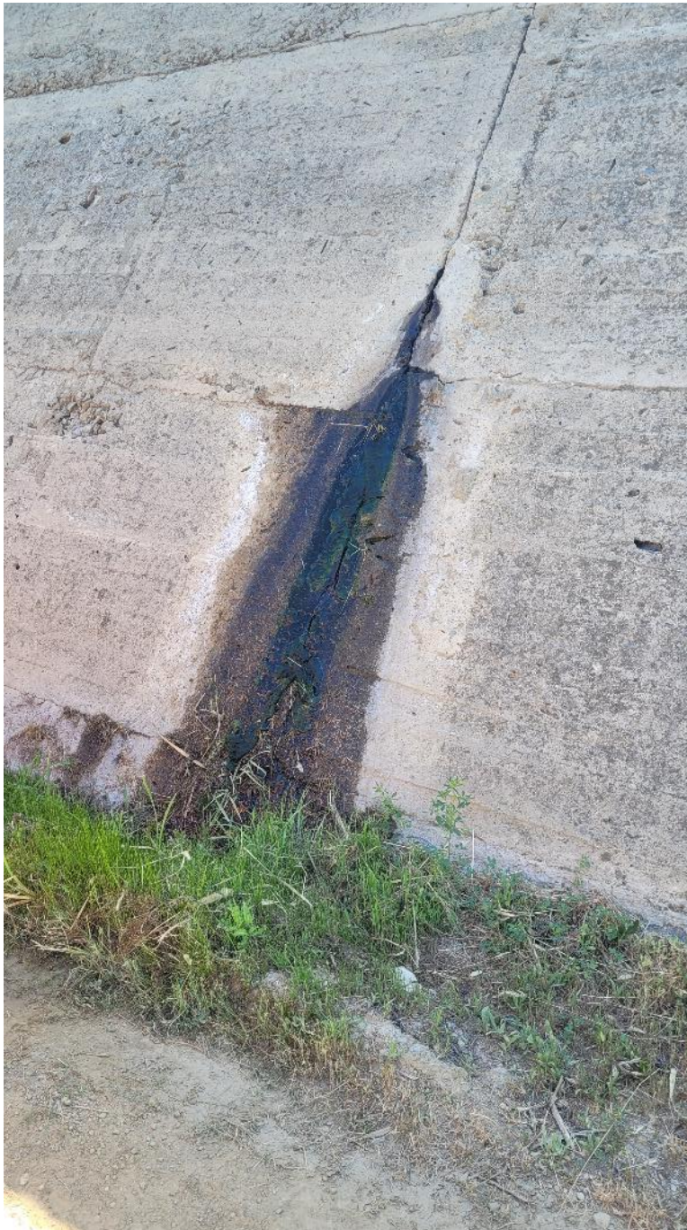
Photo 1: View of the typical seepage at the auxiliary ridge dam section at Sta. 0+68.
