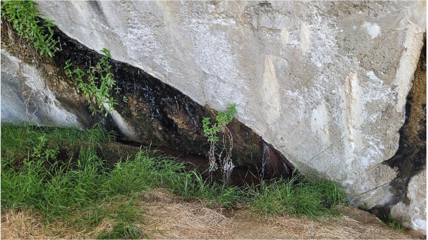
Photo 3: View of typical seepage through the multiple arch dam section.
