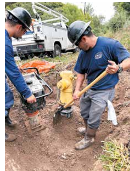
MWD staff replacing an aging hydrant, one of more than 880 public fire hydrants district-wide (courtesy photo)
