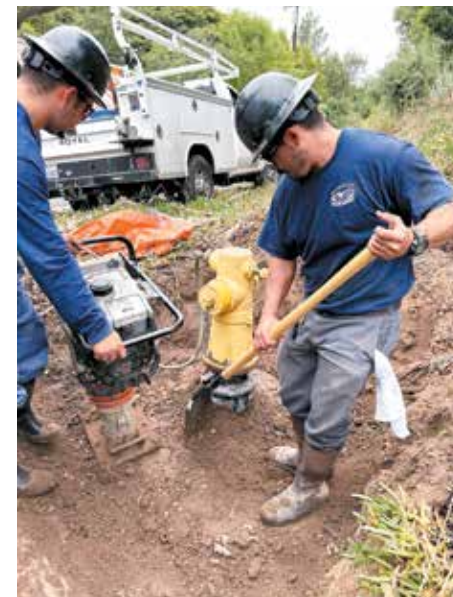
MWD staff replacing an aging hydrant, one of more than 880 public fire hydrants district-wide (courtesy photo)
