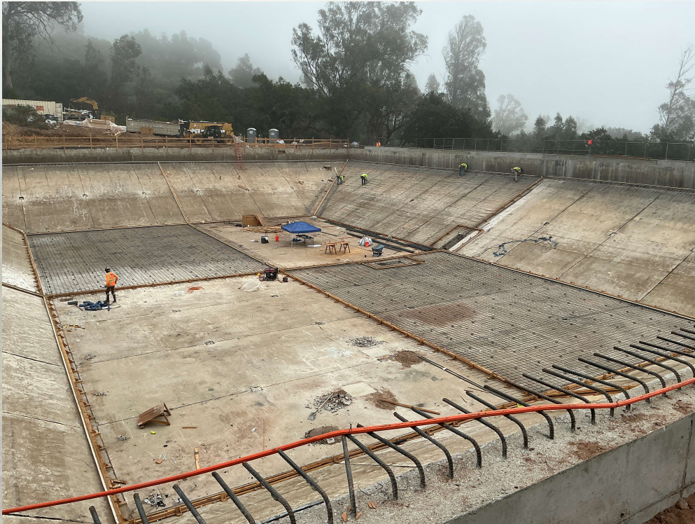
Slab Mat Reinforcement Installation
