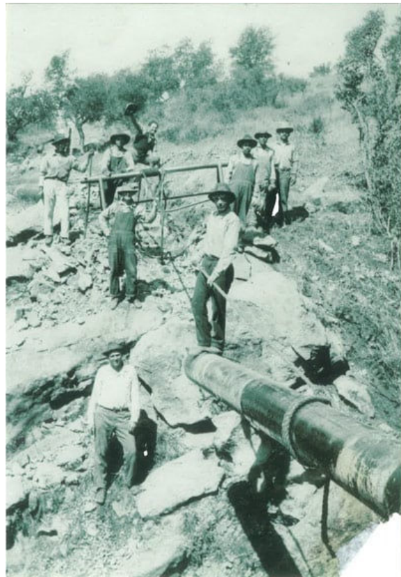
District pipeline construction, circa 1930
