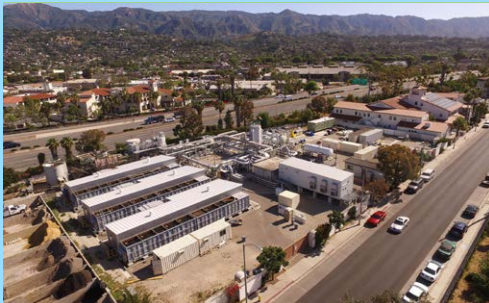
Water Supplied by the City of Santa Barbara, secured by Charles E. Meyer Desalination facility.
