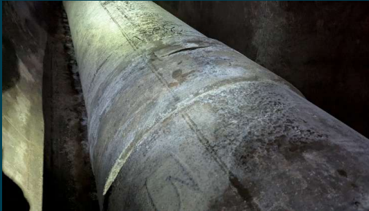
Type 1: Good condition
