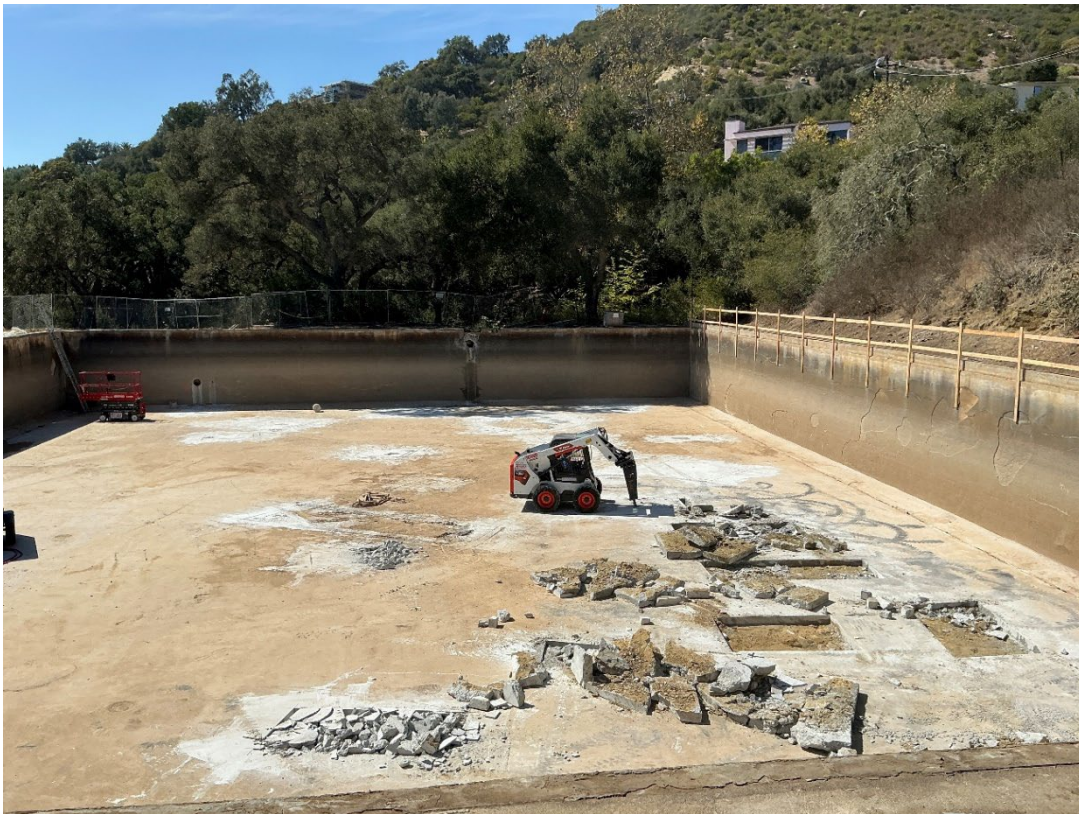
Figure 1 – Park Lane Reservoir Void Remediation Work
