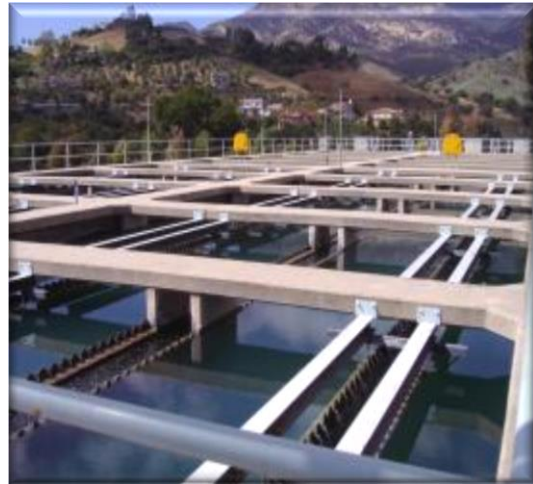
Cater Treatment Plant
