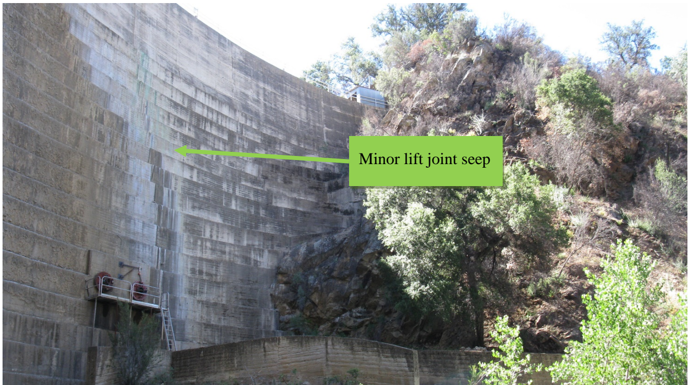
Arch Section – Downstream Face
