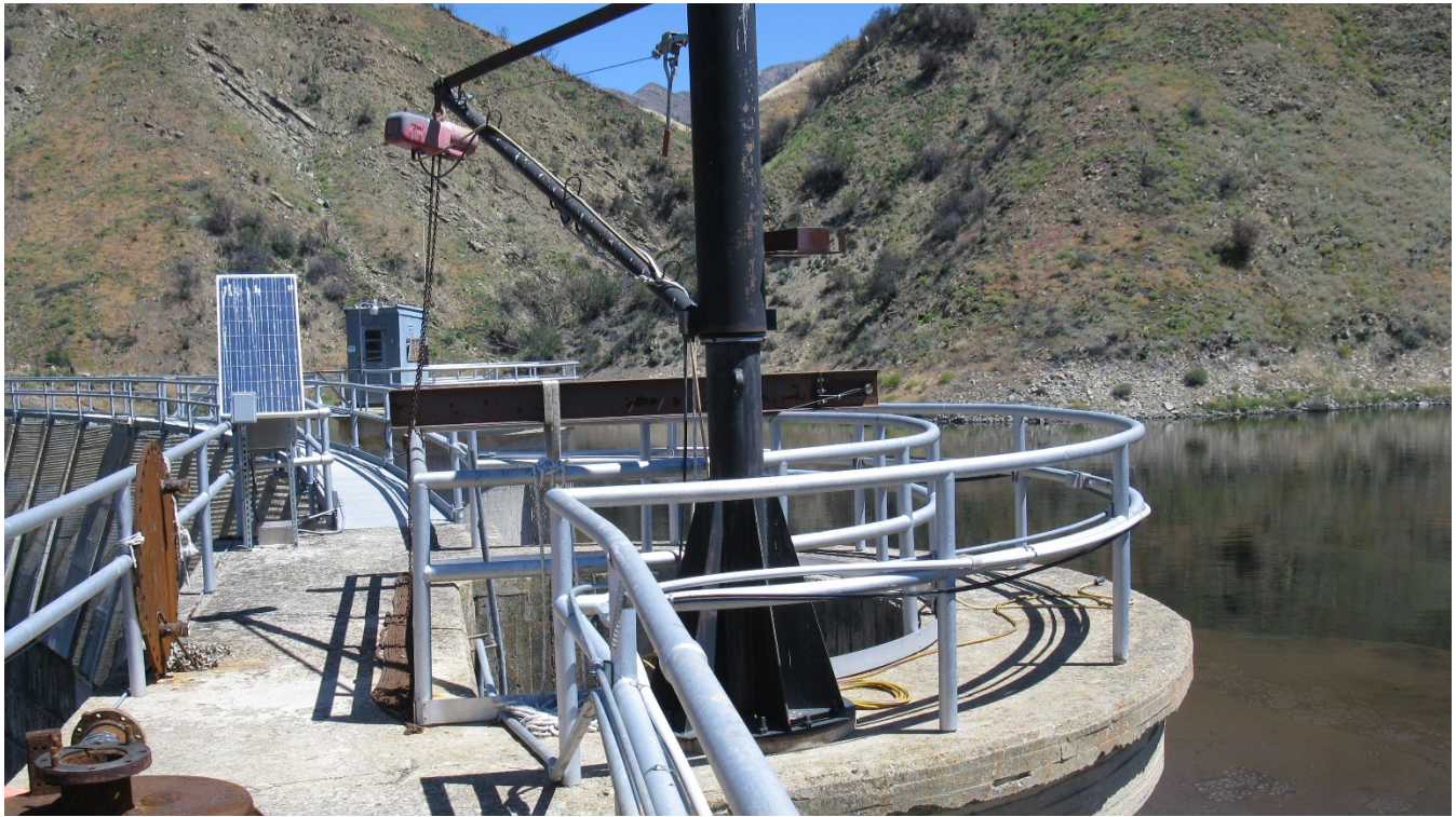
Arch Section – Crest and Outlet Towers
