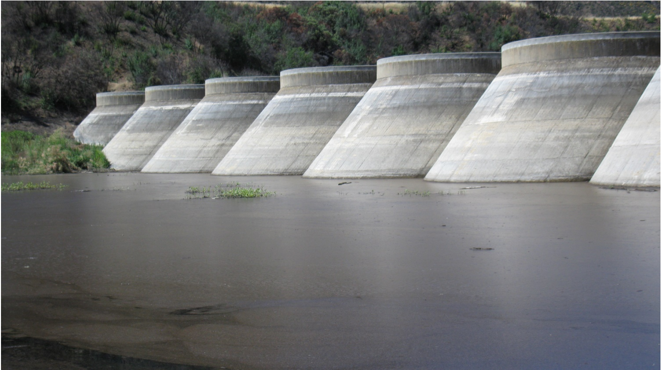
Multiple Arch Section – Upstream View
