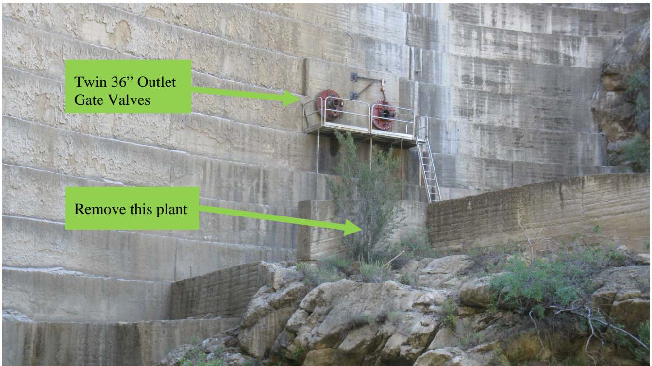
Arch Section – remove the small tree
