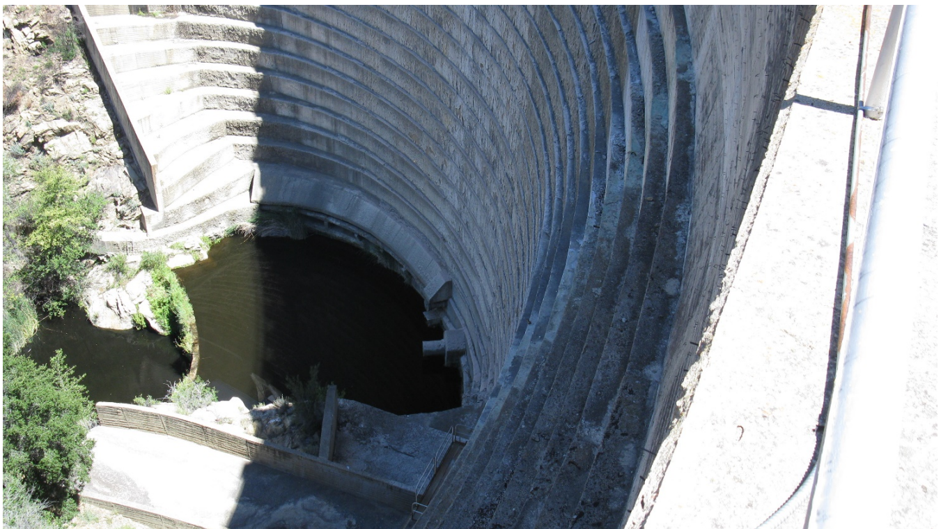
Arch Section – downstream face of spillway and plunge pool below
