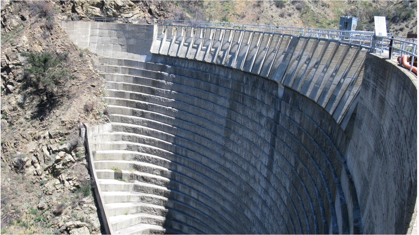
Spillway over the main dam (arch section)
