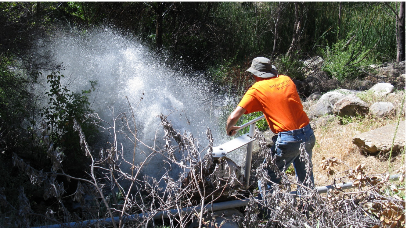
Cycling the 18-inch Blowoff Valve
