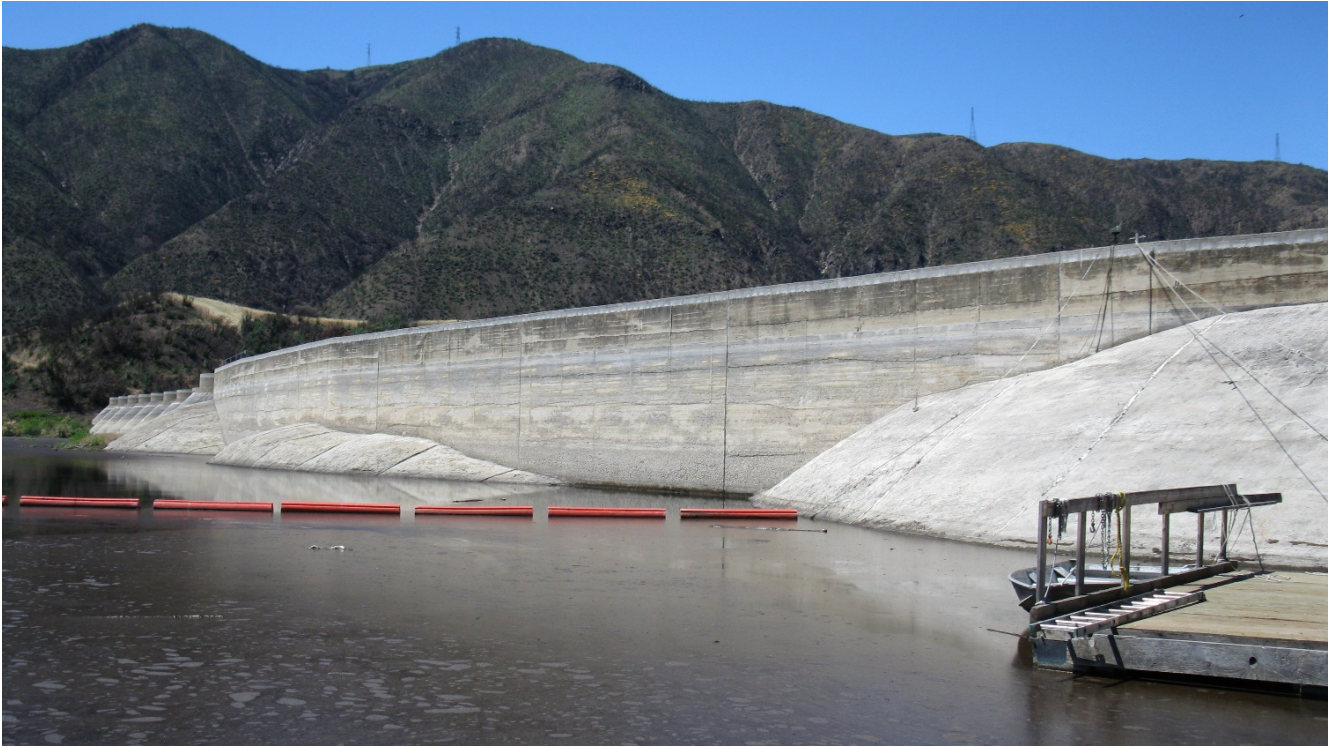
Gravity Section – Upstream Face
